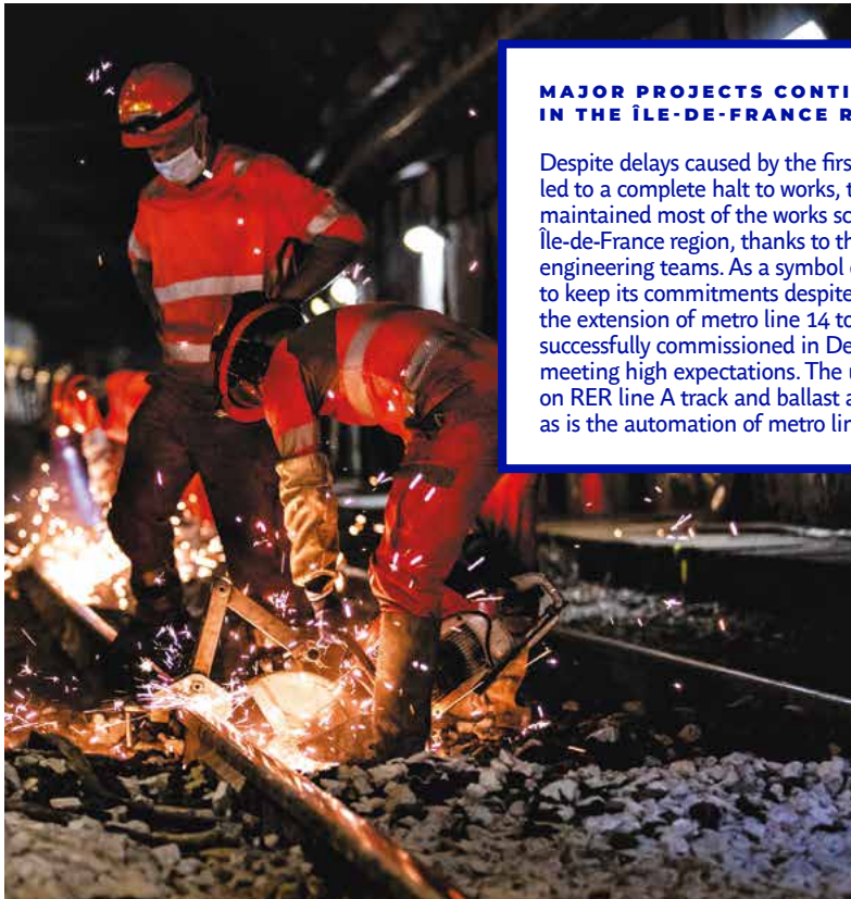
Track and ballast renewal works on RER line A in August 2020.
